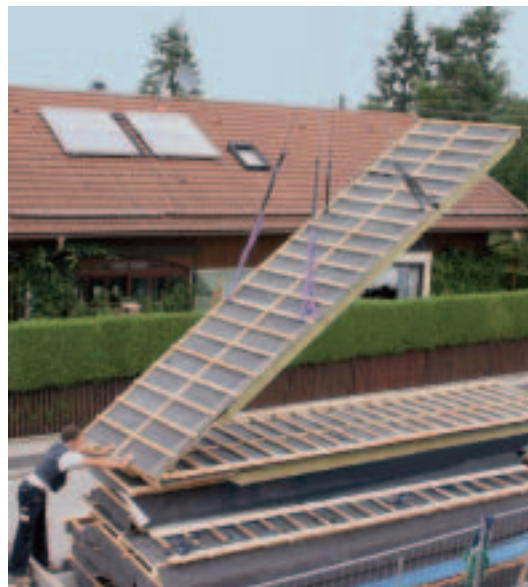
Montage Finnroof-Elemente
