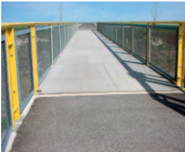
Brücke in Crailsheim
